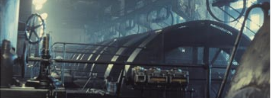
Briquetting machines at Knappenrode Briquetting Works
