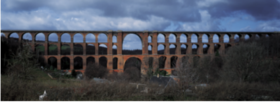
Brick built railway-bridge across the Göltz-Valley (build 1845/51)
